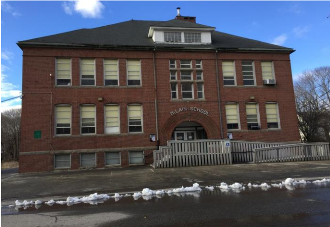
McLain School, Front entrance, East Side
